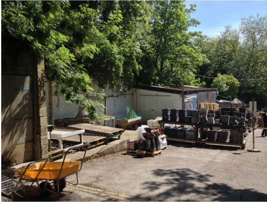
Existing brick structures used for storage
